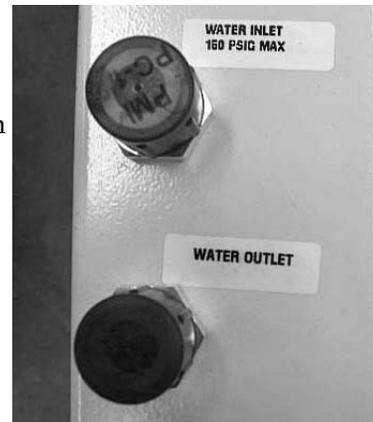
Figure 5-2. Inlet/Outlet Fittings
